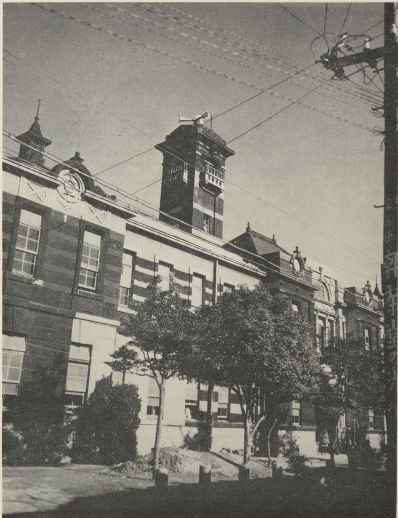
Photo 15. Fire watchtower, Nagasaki City Hall.
